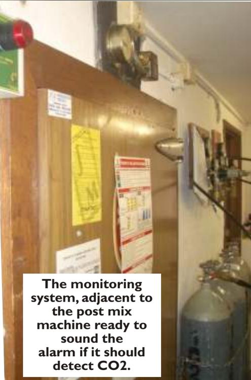
**The monitoring system, adjacent to the post mix machine ready to sound the alarm if it should detect CO2.**
